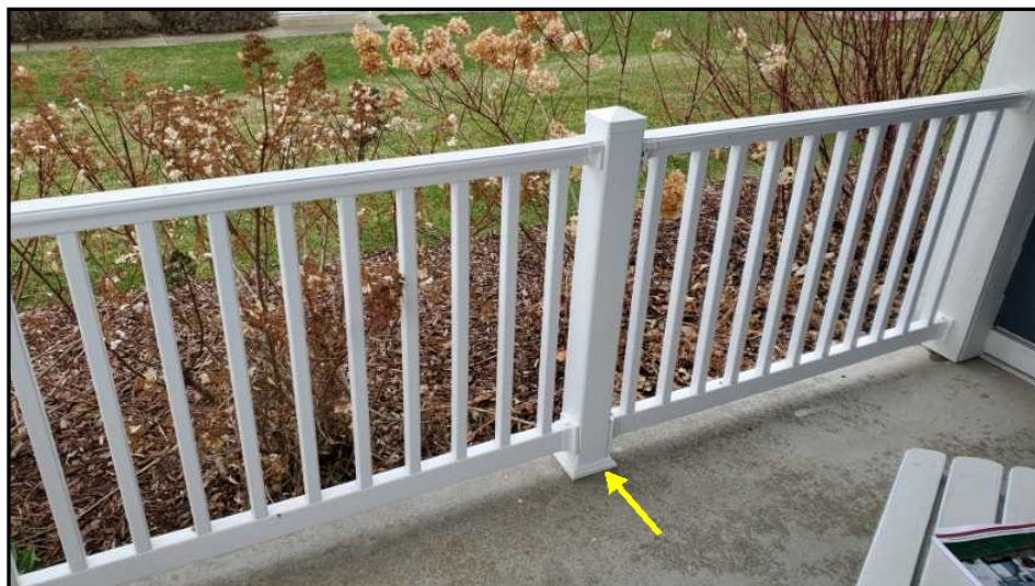
Guardrail loose
