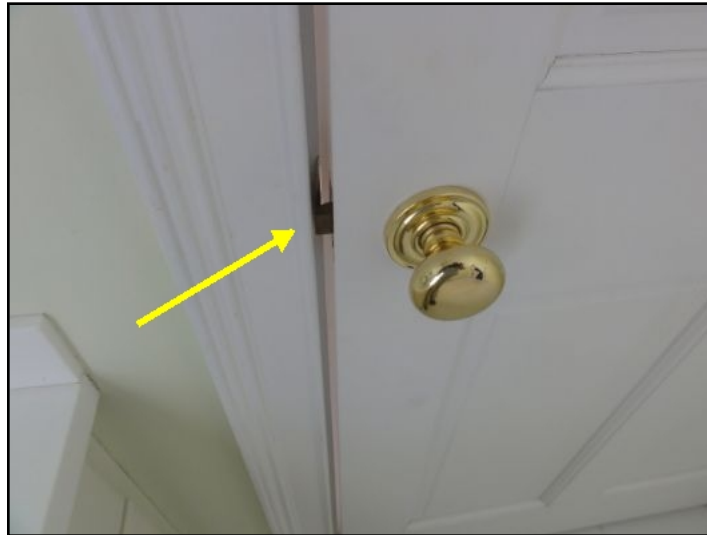
Strike plate needs adjustment to latch door
