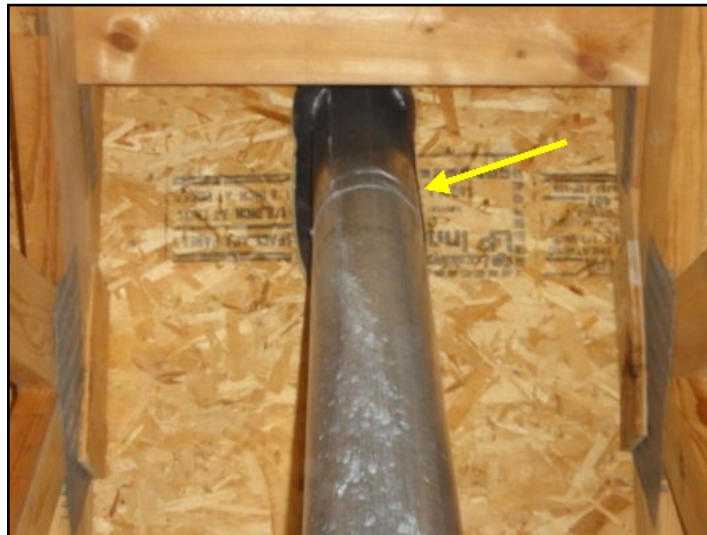
B-vent not maintaining 1" clearance
