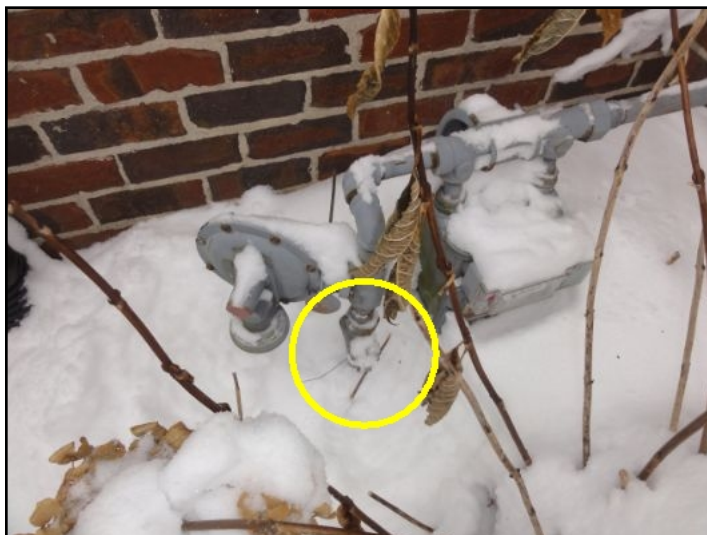
Main gas shutoff valve
