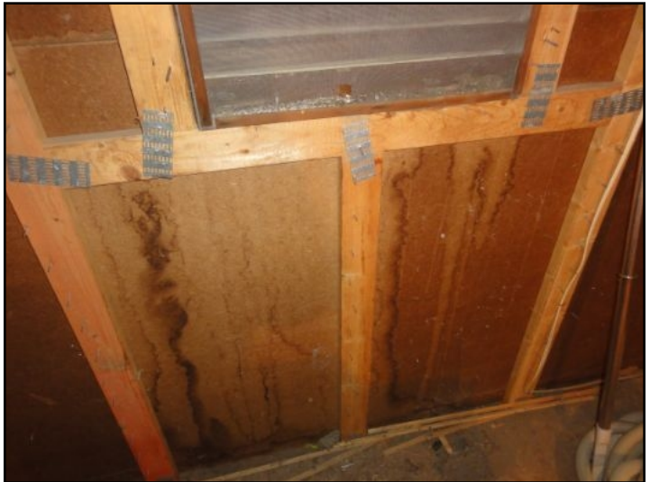
Garage attic moisture staining below gable vent
