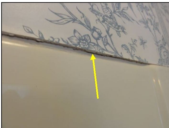
Caulk needed at shower enclosure to wall board
