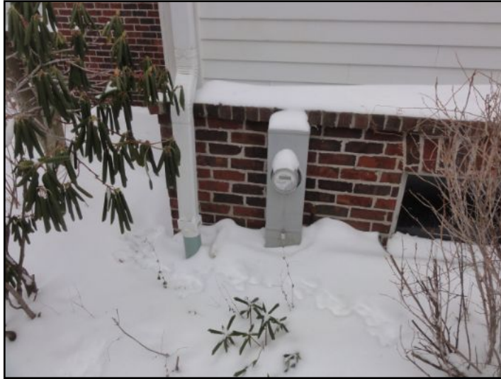
Underground electric service
