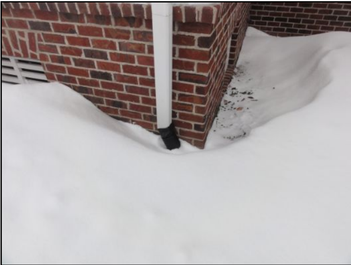
Down spouts discharge underground
