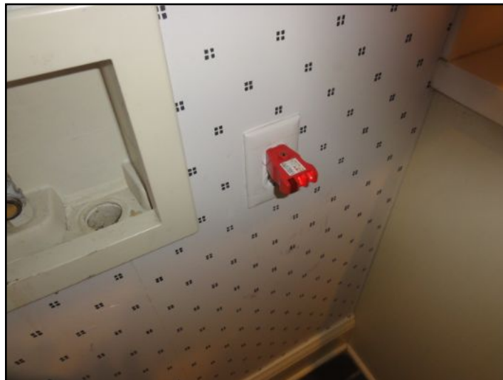
Recommend GFCI protected outlet for washer
