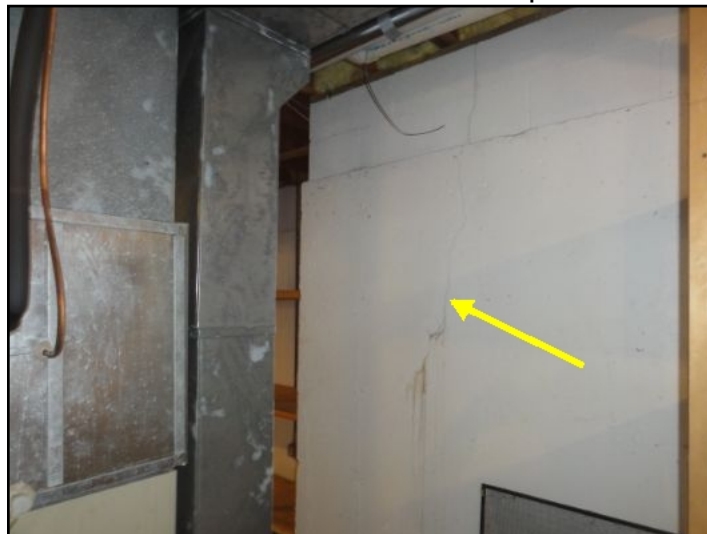
Crack in foundation wall
