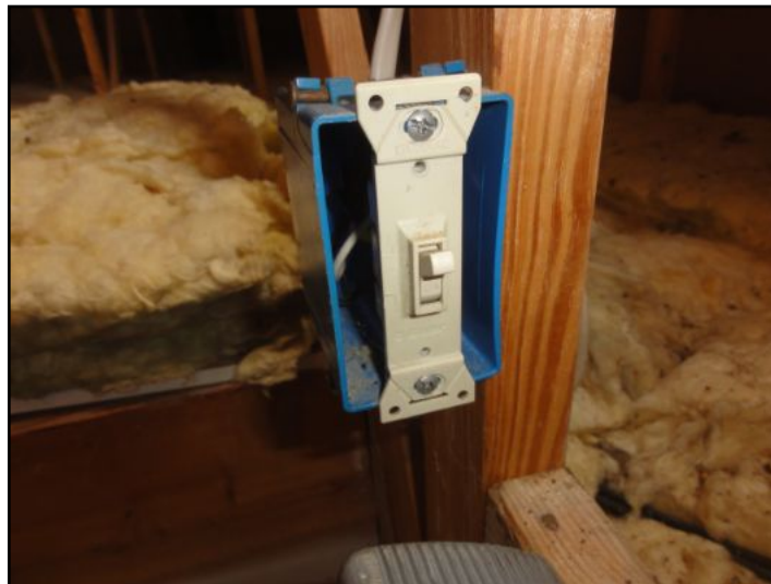
Missing switch plate
