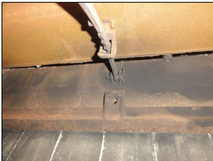
Gas fireplace has closeable damper
