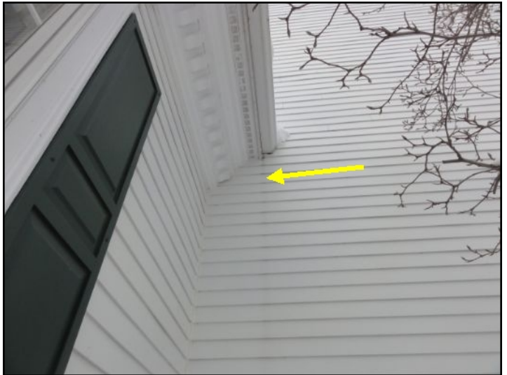
Gutter leaking down siding
