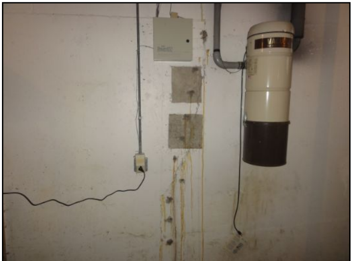
Repaired crack in foundation wall
