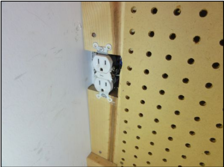
Missing outlet plate
