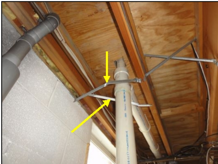
Floor joist braces removed
