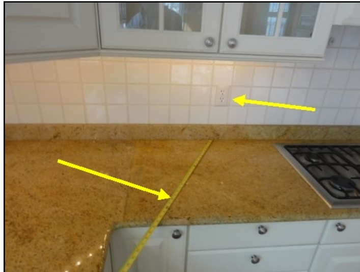
Non-GFCI protected outlet within six feet of sink
