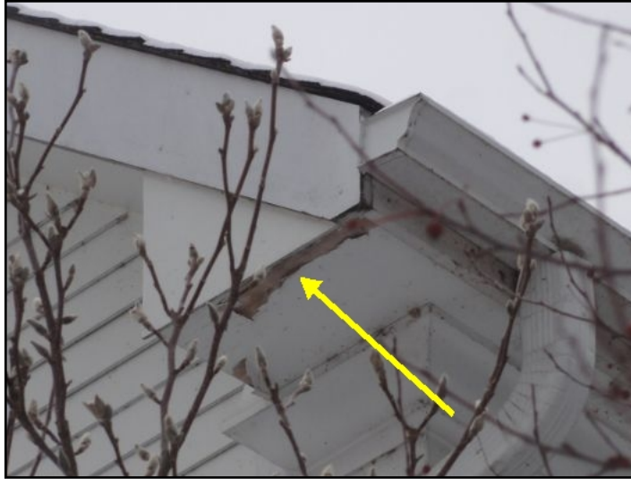
Peeled paint on soffit
