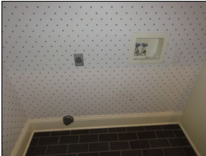
Plumbing connections for washer
