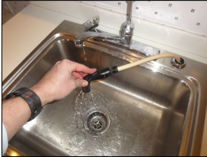
Wand doesn't shut off
