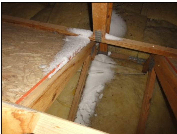
Snow blown through ridge vent
