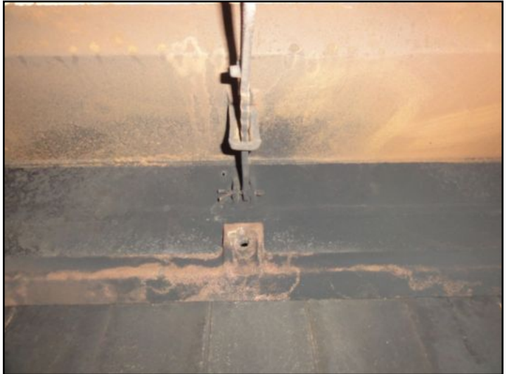
Closeable damper in family room gas fireplace
