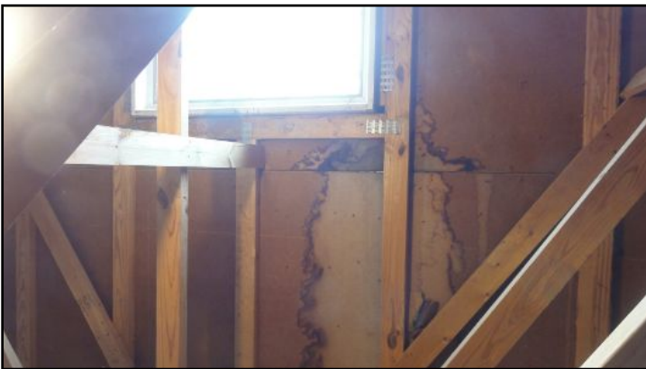
Moisture stains below attic window
