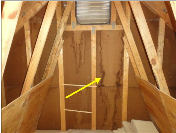
Moisture staining in attic
