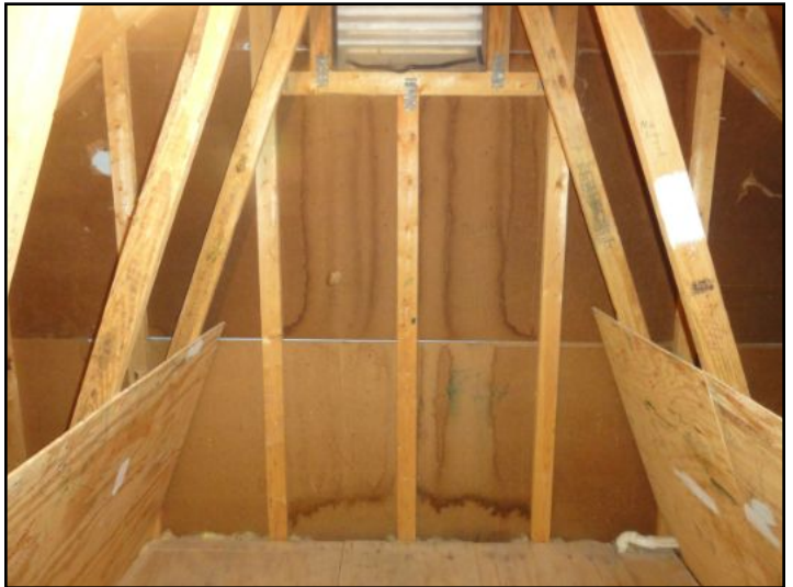
Moisture staining in attic
