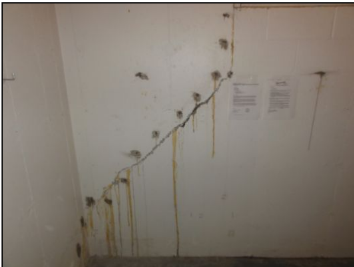
Repaired crack in foundation wall
