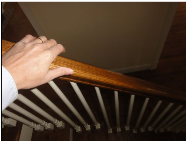
Handrail for stairway to upper level loose
