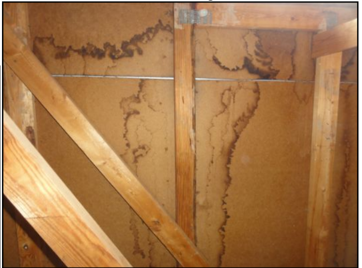
Moisture stains below attic window
