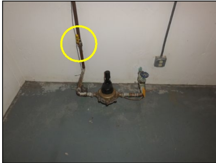
Main water shutoff valve
