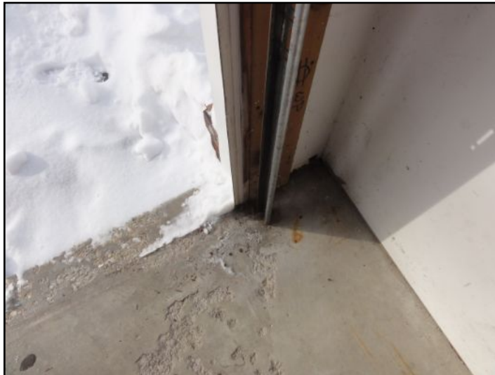
Photo sensors not installed
