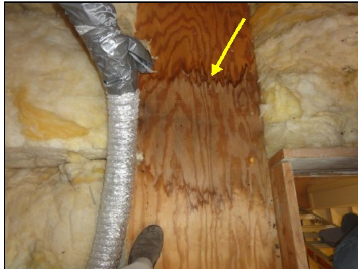
Condensate leaking out of bath vent pipe
