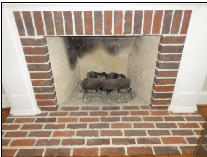
Gas fireplace appears to have gas shut off.
