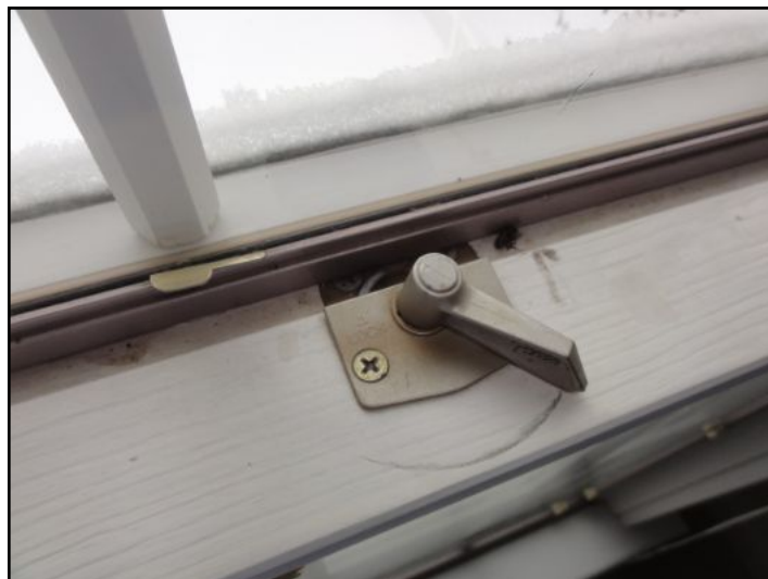
Three windows in master bedroom don't lock properly
